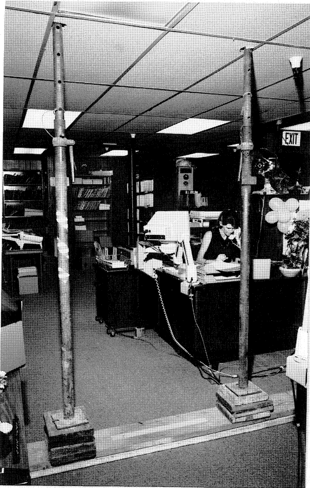
Photo 1: Structural supports in the boards's office space
